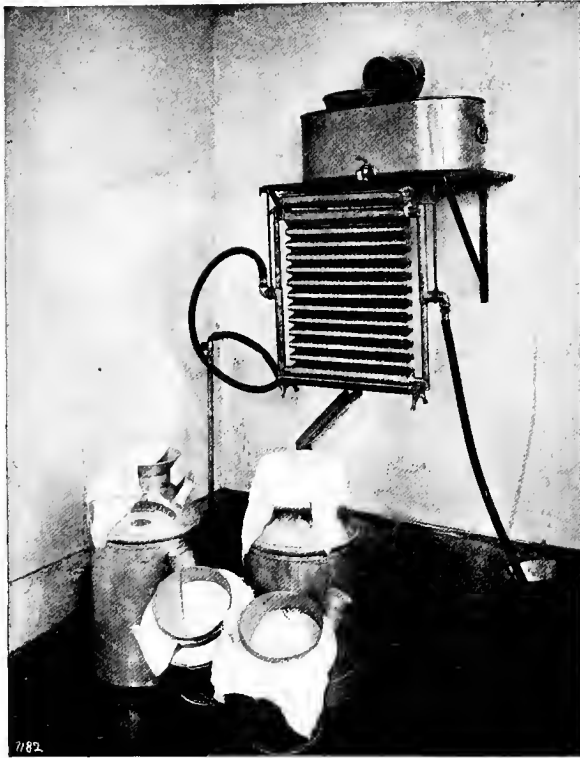
FIG. 14.—APPARATUS FOR COOLING MILK.
